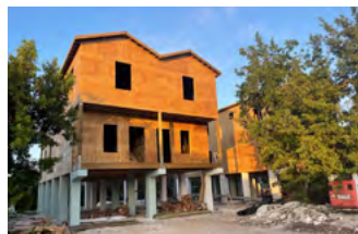
Construction progress on last four units at Moss Landing from September-December, 2022
