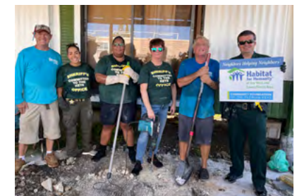
Habitat's Construction Team, Dan Livingston and Curtis Barlow, work with staff from the Monroe County Sheriff's Office on home repair jobs in Big Coppitt and Stock Island.
